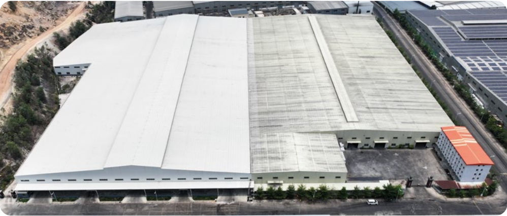
Sihanoukville, Cambodia Sihanoukville, Camboya 柬埔寨工厂
